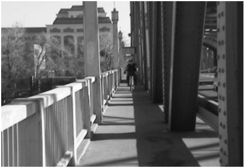
Looking east, north side of Tower Bridge
