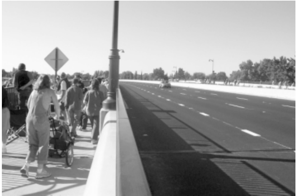
Temporarily crowded sidewalks, uncrowded road on Watt Avenue Bridge Photo by Walt Seifert
