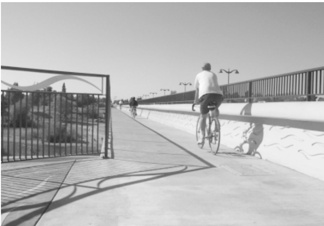
Wider sidewalk/path on Watt Avenue Bridge Photo by Walt Seifert
