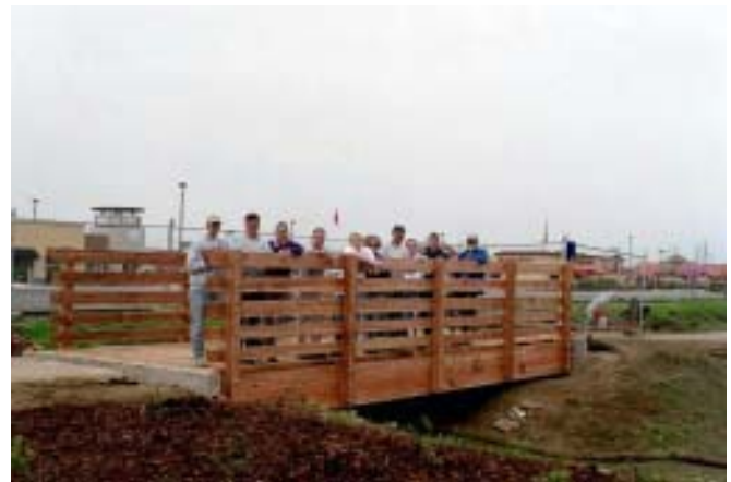
FABA Work Crew on Folsom's New Bike Bridge Photo by Tony Powers
