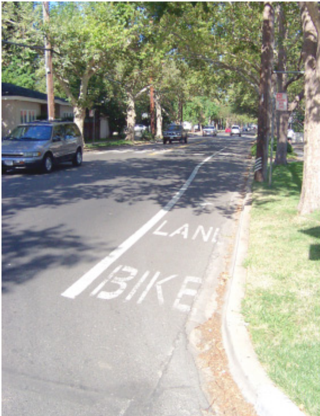
One foot gutter pan on H St
