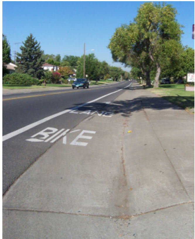
Three foot gutter pan on H St
