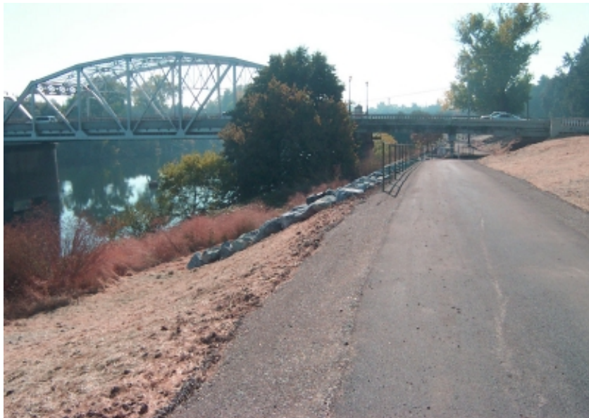
New trail under H Street Bridge
