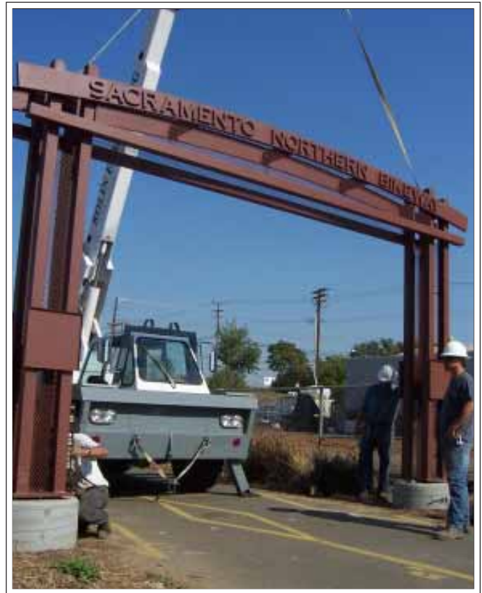
Gateway in place. Photo by Walt Seifert
