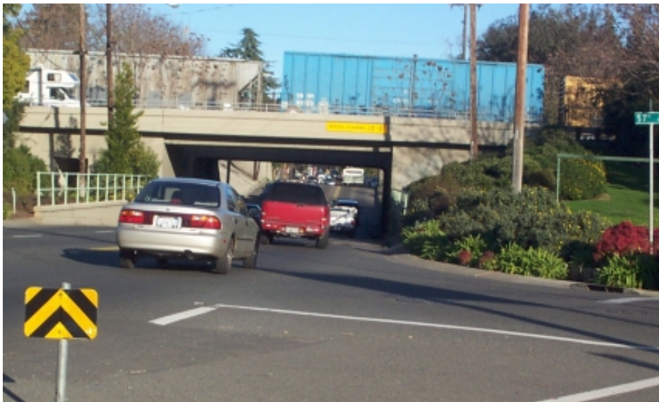
No room for bikes. H Street undercrossing of Elvas and UP tracks Photo by Walt Seifert
