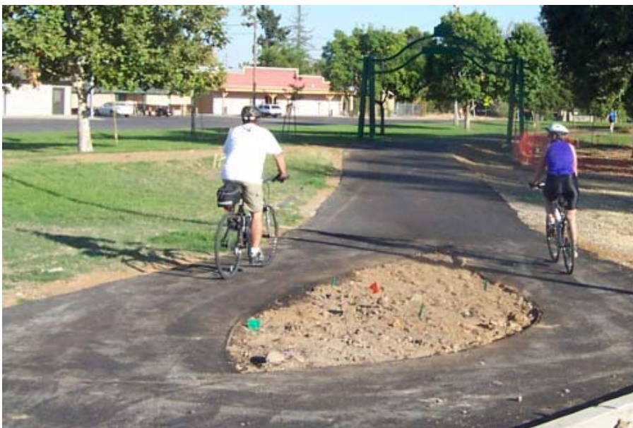
Split trail allows bollard-free entry to the Sacramento Northern Bikeway. Photo by Walt Seifert
