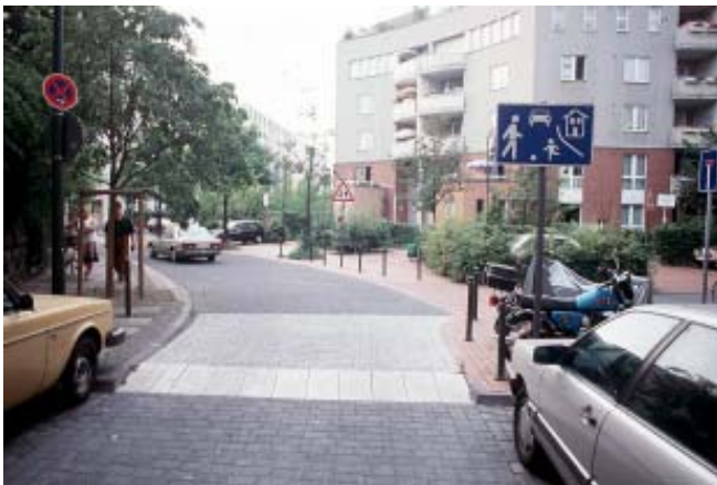
A speed table is a section of raised roadway which is a traffic calming measure. Source: Pedestrian and Bicycling Information Center
