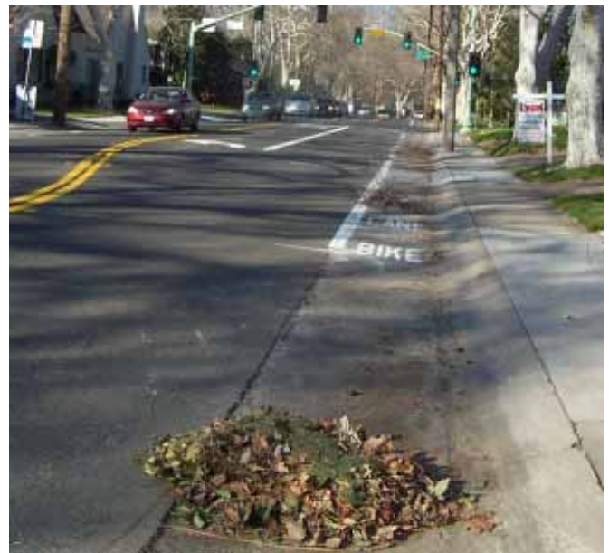
Short bike lane segment in the gutter on northbound Freeport Blvd. at 2 nd Ave. Note green waste piles in the way. Photo by Walt Seifert
