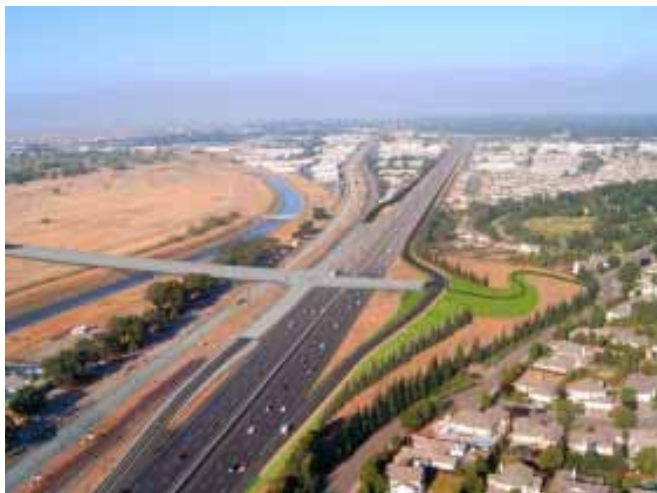
View of what Rancho Cordova Parkway interchange could look like. Image courtesy city of Rancho Cordova
